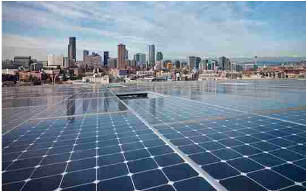
Fig.3. Bullitt Center Roof with 575 BIPV
